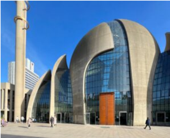
DiTiB Central Mosque Cologne, Design by Paul Böhm architects, 2006 – 2017 © Pieter van der Ree
